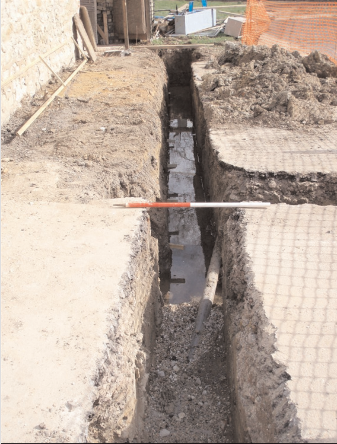
Plate 3. Close-up of service trench (facing north-east).
