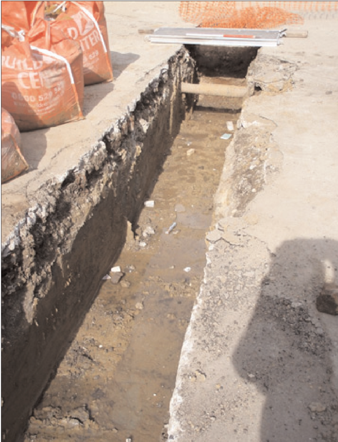
Plate 4. Close-up of foundation trenches (facing north-west).
