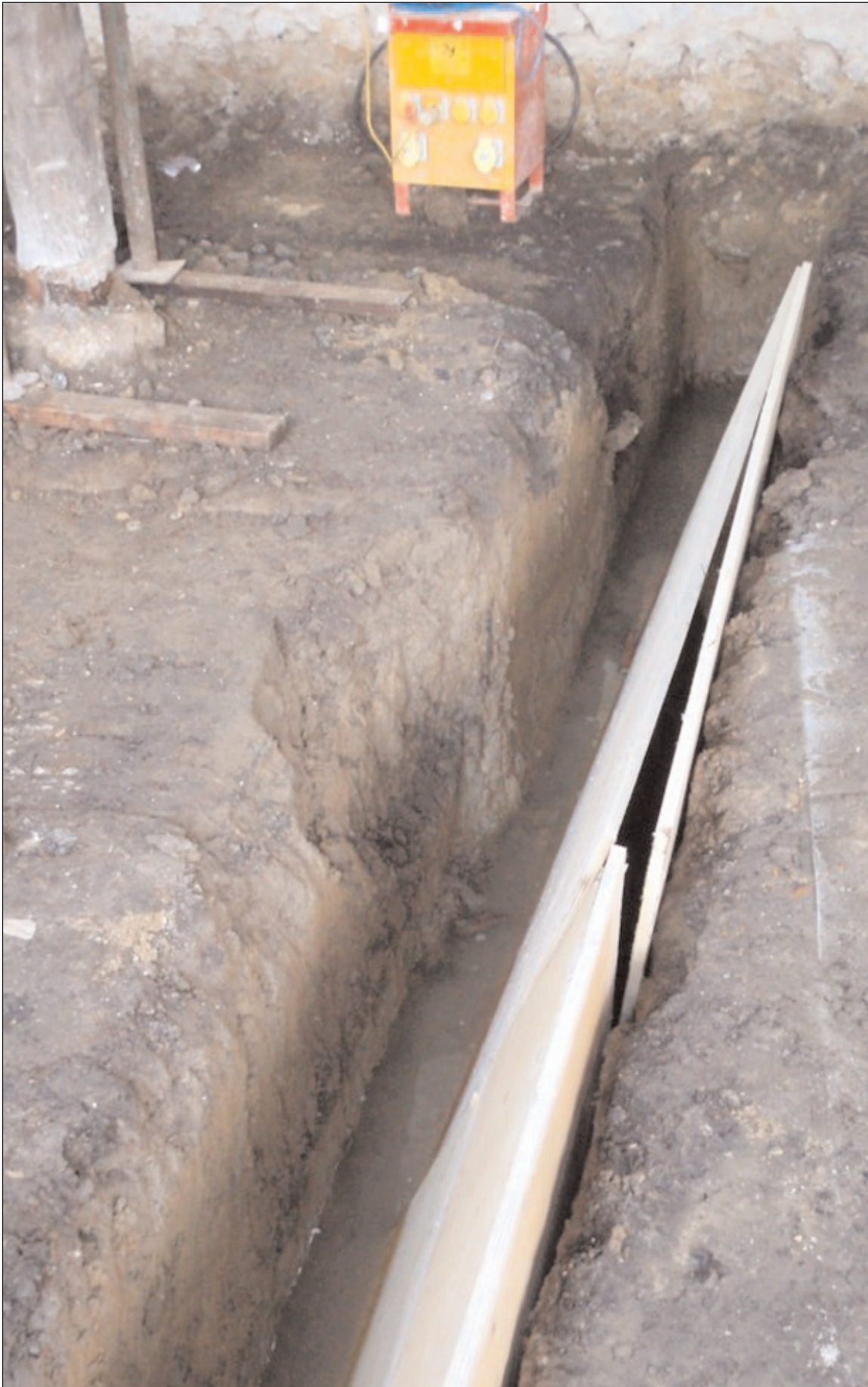
Plate 2. Showing excavated strip foundations inside granary (facing west).
