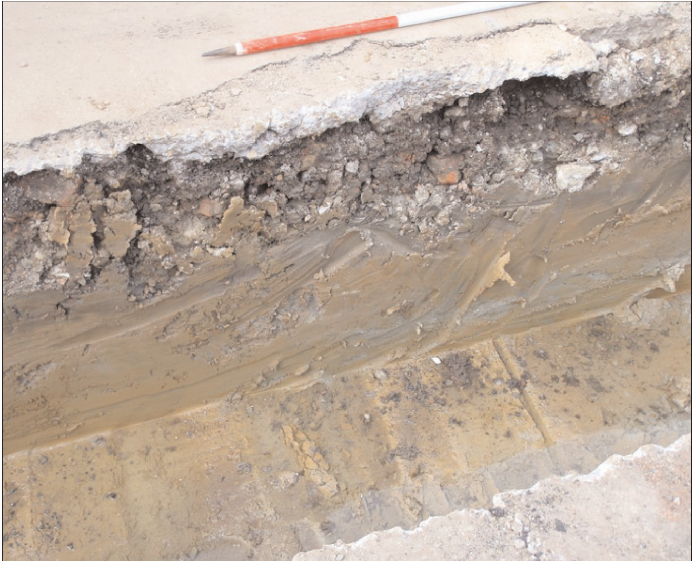
Plate 5. Close-up of foundation trenches (facing west).
